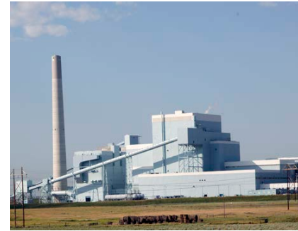
Dry Fork Station Gillette, WY
